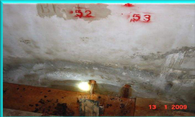
Photo No. 5: A View of a Core Hole at the Floor Slab
