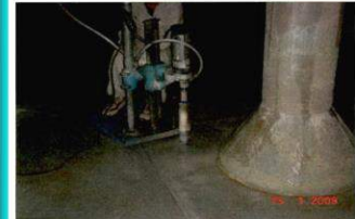
Photo No. 1: Extraction of Core from Column Footing is in Progress
