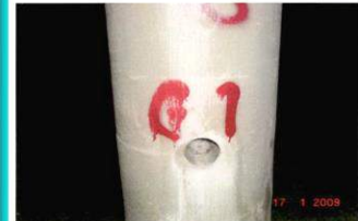
Photo No. 3: A View of the Column after Core Extraction.
