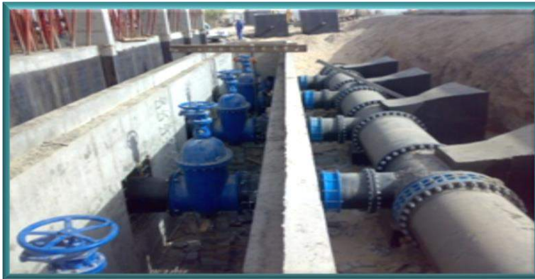
Conversion of Open Irrigation Channels into Pipelines, Al Hassa - KSA
