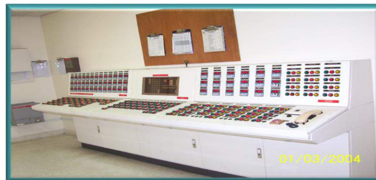
Jeddah Islamic Port - KSA
