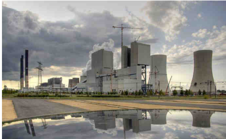
Boxberg Thermal power plant
