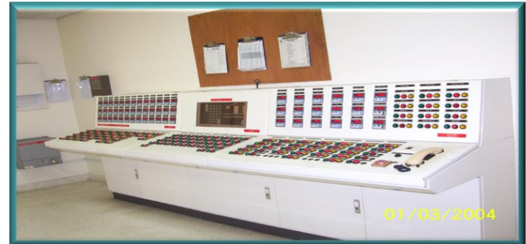
Jeddah Islamic Port - KSA
